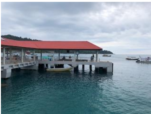
Main jetty at the village
