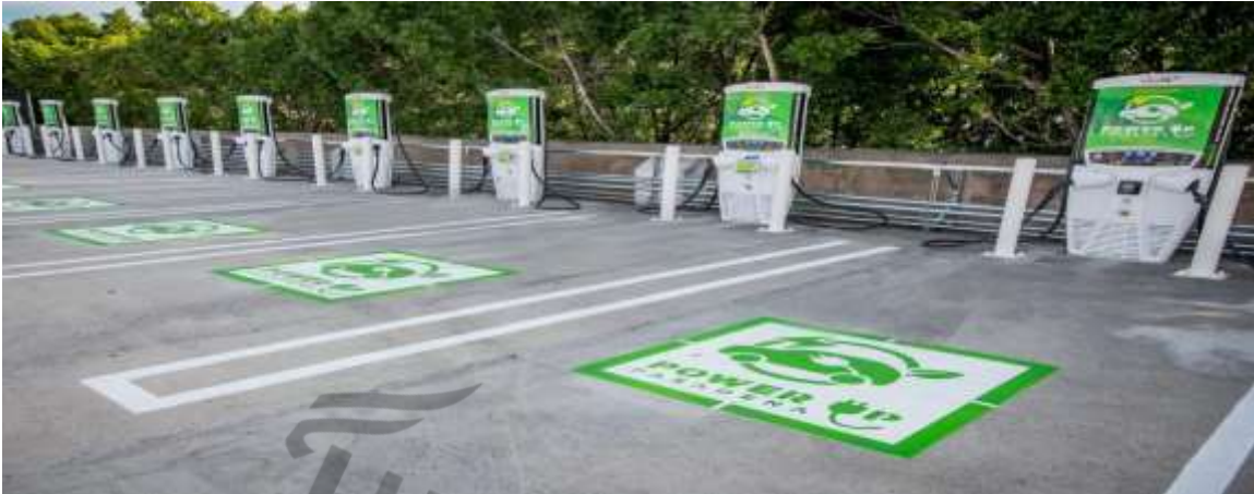
Figure 40. Example Electric Vehicle Charging Station Facility
